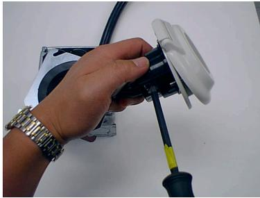
5. Back off terminal screws on the rear housing of the inlet. Insert wires into color coded openings on the back of the inlet. Tighten terminal screws to 14-20 in.-lbs. torque. **Make certain there is no wire insulation under any terminal.**
