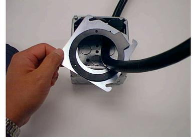
3. Pull out enough of cable to allow room to work. Tighten two screws of the box extender to the box with 10-12 in.-lbs. Feed cable through box cover opening and rubber inlet mounting gasket.
