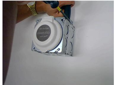
6. Position the gasket and inlet over the box cover opening, align the mounting holes and attach the inlet with provided 8-32 screws. It may be necessary to pull cable back out of the box through the strain relief to prevent wires from crowding. Fasten the box cover to the box extender and tighten the strain relief to 12-16 in.-lbs. torque.
