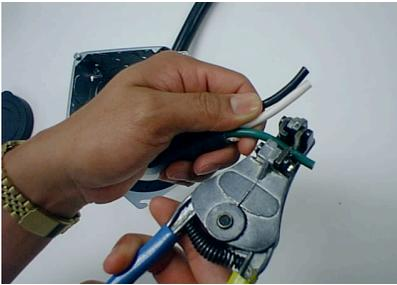
4. Remove 2" outer cable jacket. Strip wire ends 1/2" to 5/8". **Make sure the wire strands are clean and not corroded.** If necessary, cut back the wire until clean wire is uncovered. **Do not solder the ends of the wire.**
