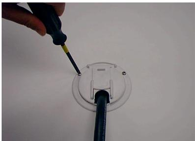
1. Remove existing mouse hole plug housing by unscrewing three mounting screws. Pull out and cut off cable leaving enough cable from the mounting hole to work on (approximately 12 to 18 inches).
