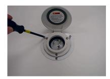
**6.** Position the gasket and inlet over the adapter mounting bracket. There are two brackets provided. Choose the appropriate mounting bracket based on the size of the hole. Align the mounting holes and tighten the screws to 5-7 in.-lbs. torque with provided 8-32 screws. Fasten the mounting bracket to existing mounting holes.
