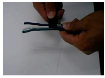
2. Remove 6" outer cable jacket and fillers. Use electrical tape to cover the jacket and flatten out conductors, leaving 2" exposed conductors. Feed the cable through the large neoprene gasket and adapter mounting bracket. Insert the conductors through the rear safety enclosure.
