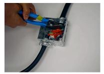
**1.** Unscrew J-box cover and cut off all wire connections
