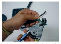
4. Remove 2" outer cable jacket. Strip wire ends 1/2" to 5/8". Make sure the wire strands are clean and not corroded. If necessary, cut back the wire until clean wire is uncovered. Do not solder the ends of the wire.
