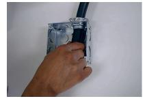
2. Unscrew strain relief to release cable grip. It may be necessary to replace with provided strain relief. Pass the cable through strain relief and box extender.
