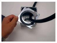
**3.** Pull out enough of cable to allow room to work. Tighten two screws of the box extender to the box with 10-12 in.-lbs. Feed cable through box cover opening and rubber inlet mounting gasket.
