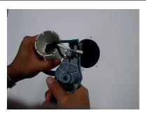
3. Strip wire ends 1/2" to 5/8". Make sure the wire strands are clean and not corroded. If necessary, cut back the wire until clean wire is uncovered. Do not solder the ends of the wire.
