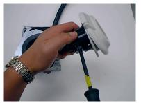
5. Back off terminal screws on the rear housing of the inlet. Insert wires into color coded openings on the back of the inlet. Tighten terminal screws to 14-20 in.-lbs. torque. Make certain there is no wire insulation under any terminal.
